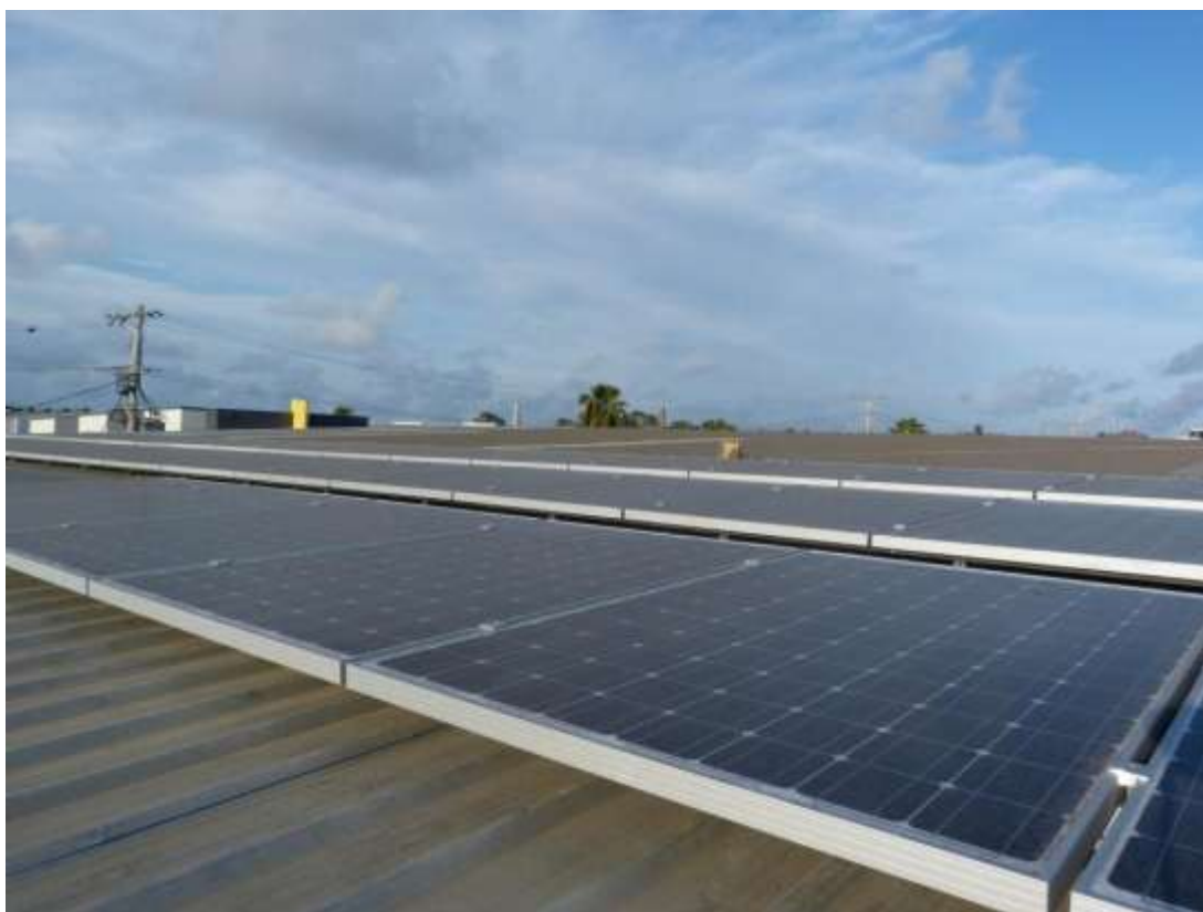
10kW Solar panel system, 84 Hanson Road workshop roof.
