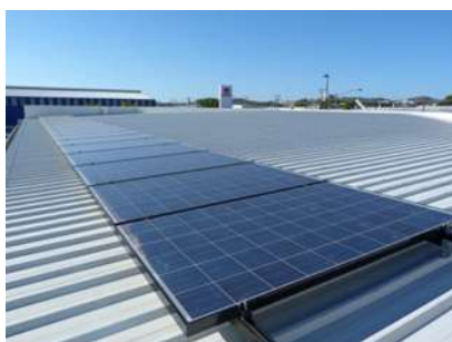
5kW solar panel system, 84 Hanson Road showroom roof.
